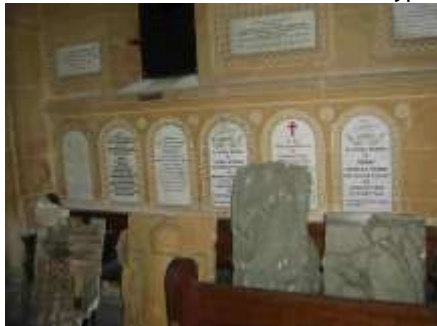
Interior west wall
