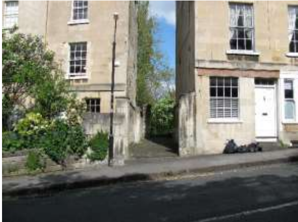
Figure 1 The entrance between 5 and 9 Lyncombe Hill
