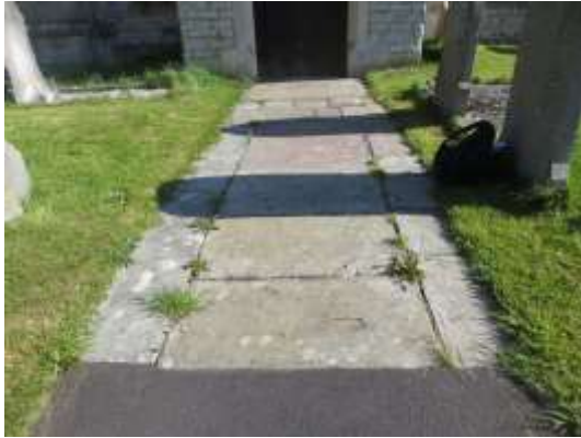
The path from the southern path to the porch is made up of a group of slabs. Two of these seem to be displaced memorials as there are faint remains of incised inscriptions.
