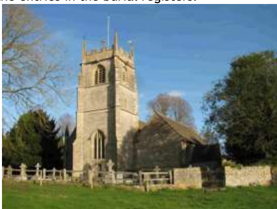
Figure 1 The church from the west
