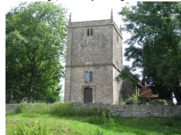
The church's tower from the west.
