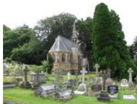
Figure 13 Eyre Chapel from the east
