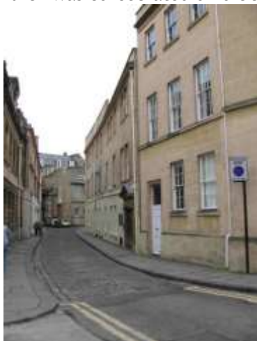
Figure 2 The façade in Old Orchard Street
