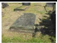
Slab with a slightly curved upper surface. Partially delaminated.
